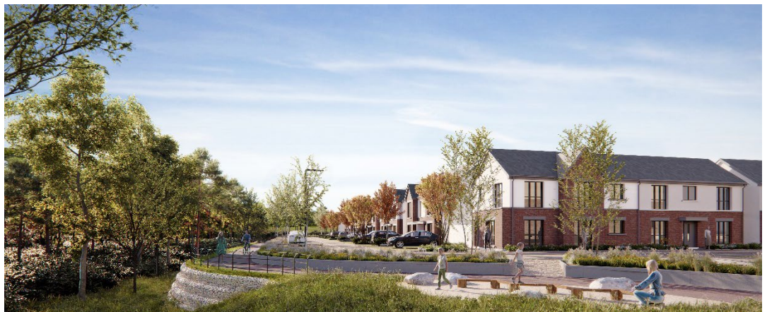
Figure 3.8 CGI Images of the Proposed Units and Green Link Running Along the Site Boundary
